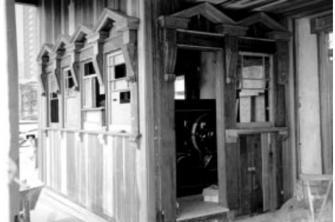
☞ ☛ Two views of Angels Flight winch house. During restoration original wooden building was completely stripped and refinished prior to fresh coating of orange and black paint.
